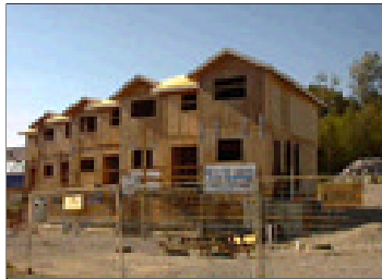
Burnaby construction site.
